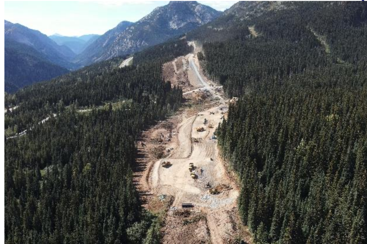
Figure 3: Preparation of Launching Platform and drilling Pad
