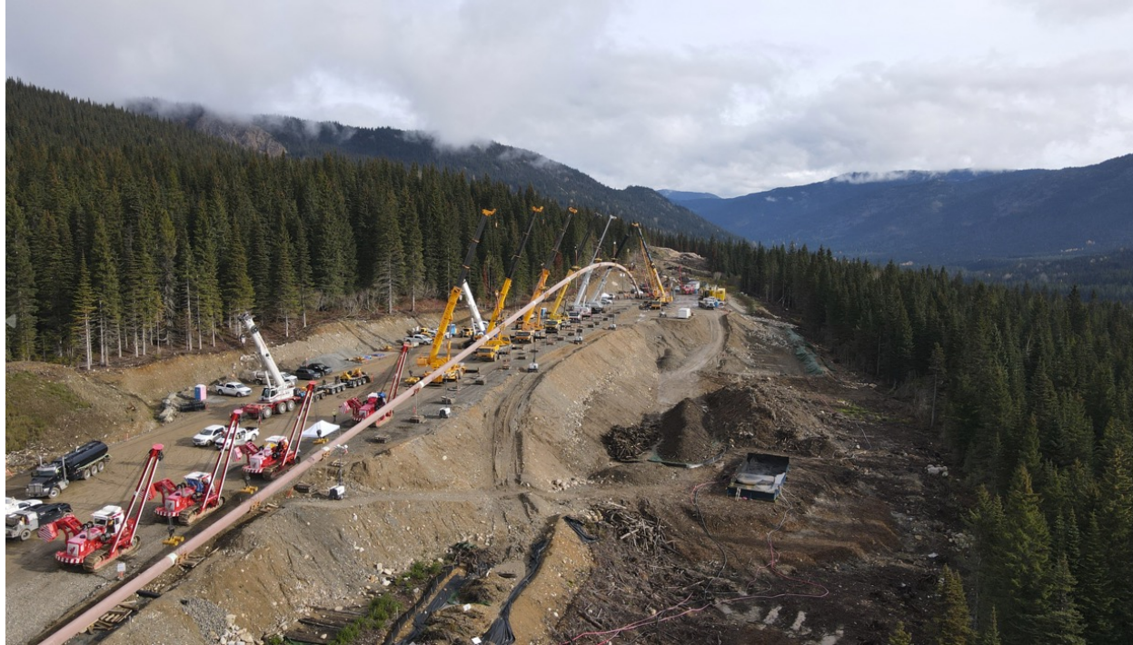
Figure 5: Pullback – Pullback execution
